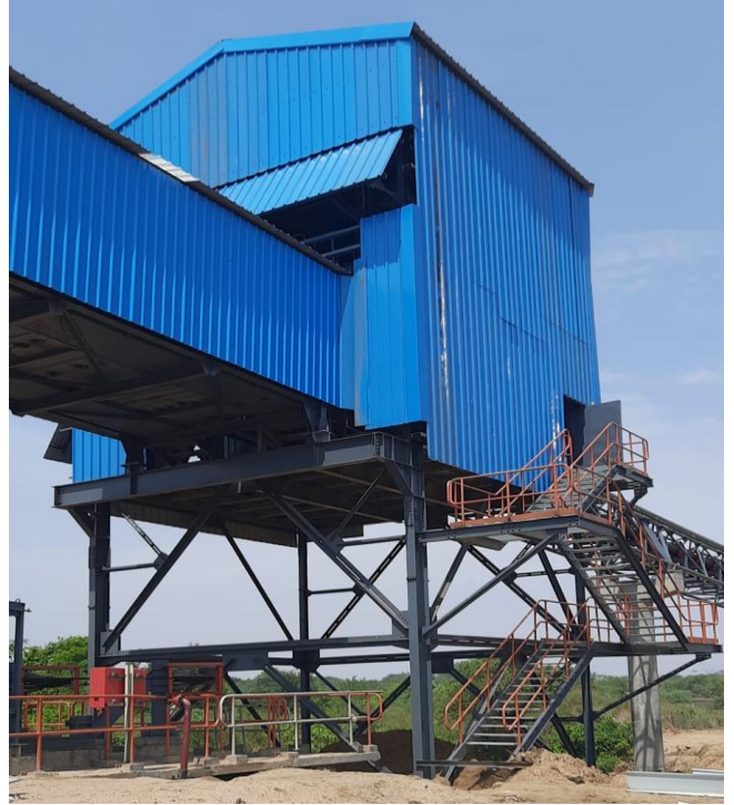
Cladding at DST-02
