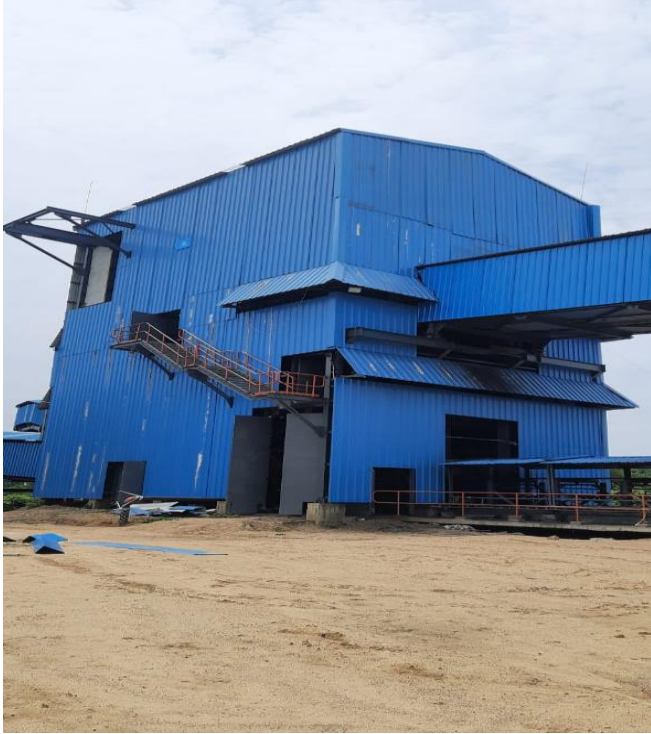
Cladding at Junction house – JH01
