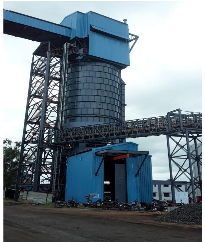
Cladding at Surge Hopper at Bhatadi
